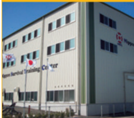
訓練棟 Training Facility
